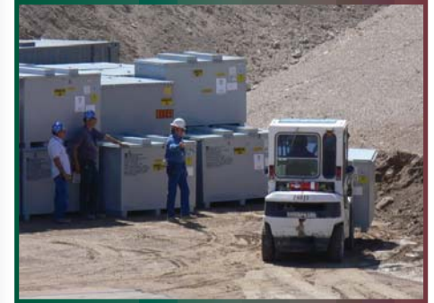
Workers place a metal box containing mixed low-level radioactive waste in a disposal cell at the Area 5 Radioactive Waste Management Complex located in the southeast portion of the NNSS.
