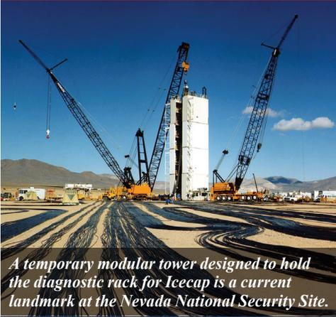
*A temporary modular tower designed to hold the diagnostic rack for Icecap is a current landmark at the Nevada National Security Site.*
